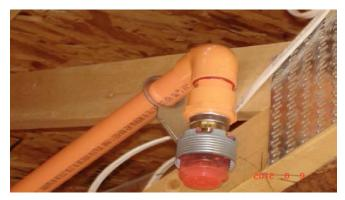
much smaller internal diameter. CPVC Installation is fast, can be easily changed or added to in the field, and is significantly less expensive than steel when you take into account the material and labor savings.
